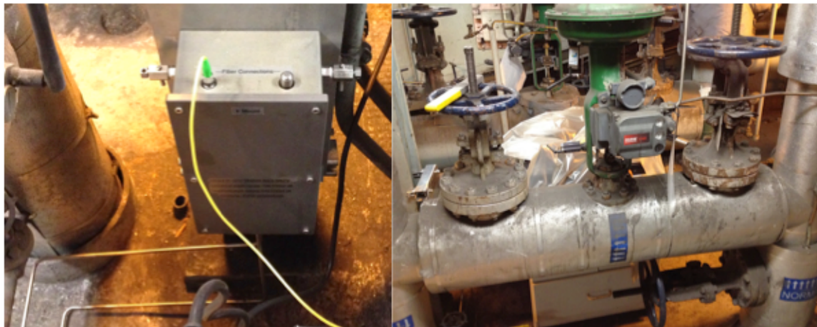
FIGURE 1: The optical fiber-based pressure sensor (left) was installed in the Penn State Steam plant as part of long-term performance testing, and measured differential pressure across a boiler feedwater valve (right).
